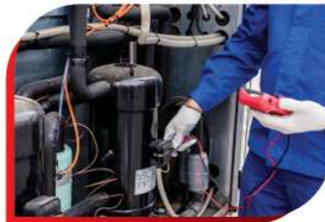
CHILLER & EQUIPMENT REPAIR WORK
