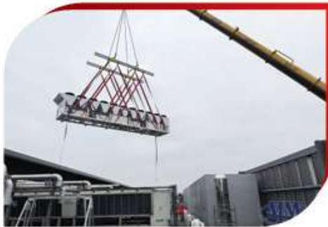
CHILLED WATER PUMP SEGMENT
